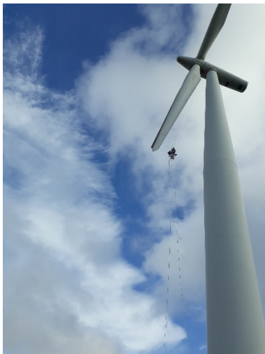
Lower off the blade until ropes are vertical
