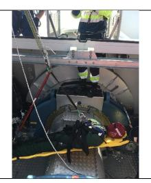
When the casualty is in the hub and secure (stretcher on the checker plate and no risk of falling off) move the pully system into the nacelle.
